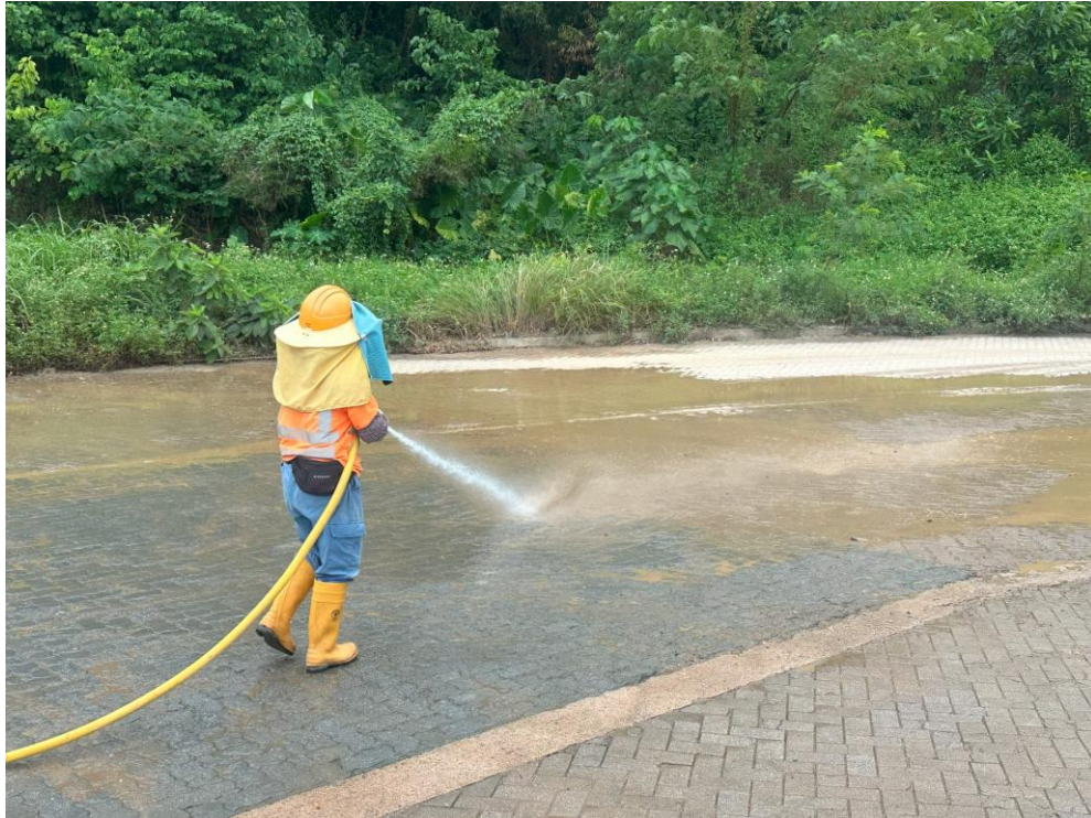
Photo 5 – Wet suppression was applied on site.
