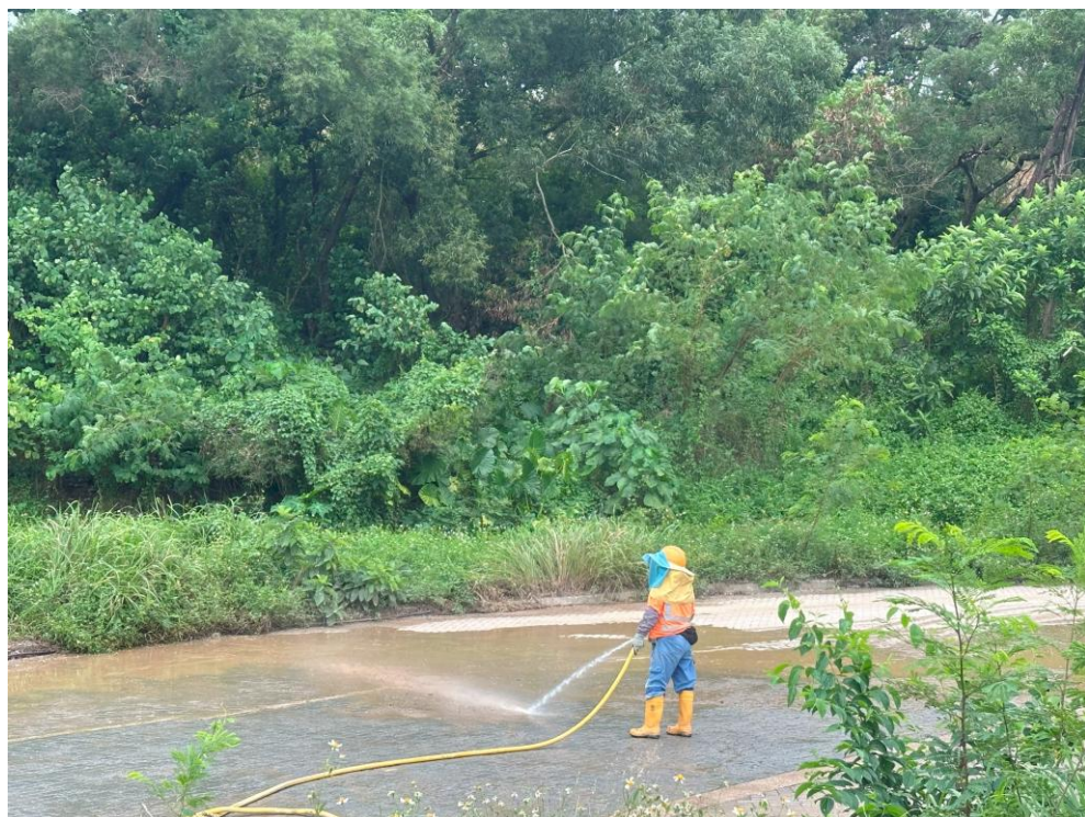
Photo 6 – Wet suppression was applied on site.
