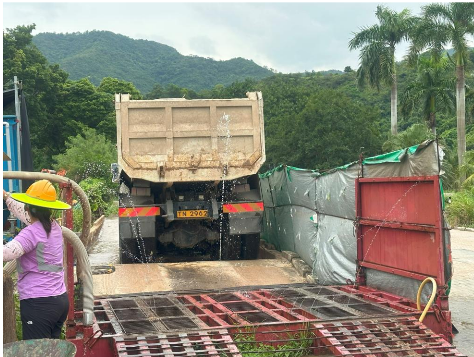
Photo 2 – Wheel washing facility provided behind site entrance.
