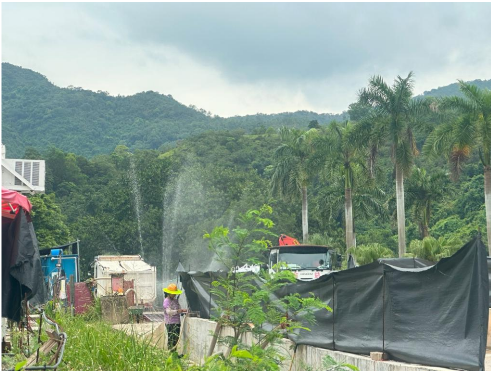
Photo 1 – Wheel washing facility provided behind site entrance.
