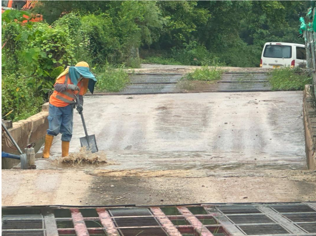
Photo 3 – Cleaning up of the heel washing facility.
